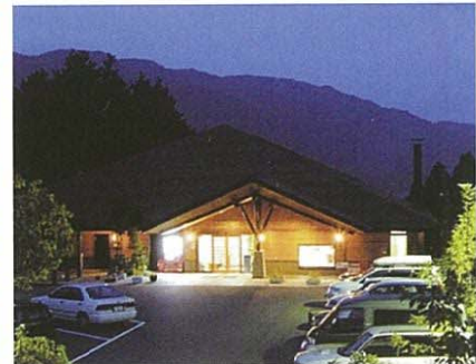
PFI project for the improvement of Togayama Hot Spring facilities (Hyogo)
