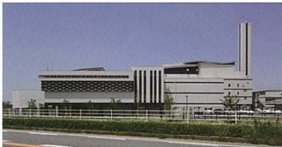
Yatsushiro City Environment Center (Incineration Facility / Recycling Center) (Kumamoto)
