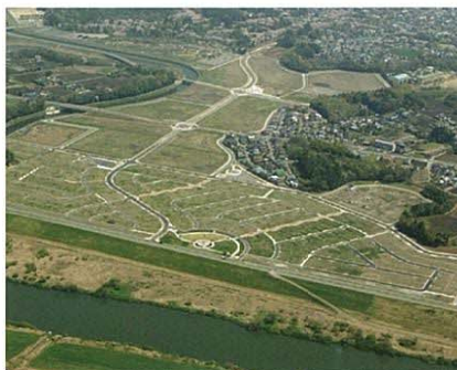
Integral land adjustment project with super levees (Chiba)
