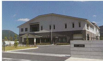
Seiyo City Sanitation Center (sludge reprocessing facility) (Ehime)
