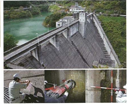
Dam inspection, maintenance and planning to prolong the service life
