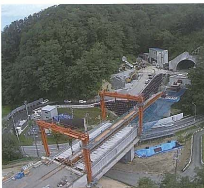
Sanriku Coastal Road Project Promotion PPP
