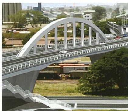
Nairobi Viaduct and Road Improvement Project (Kenya)
