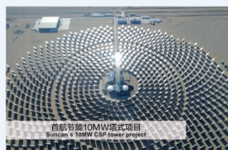
塔式太阳能光热发电 Tower Concentrating Solar Power
