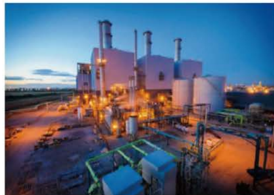
Figure 13 Saltend power plant in UK
