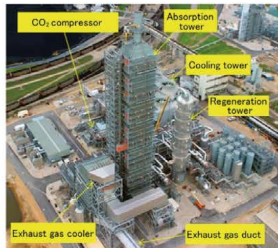
NRG Energy, Inc. and JX Nippon Oil & Gas Exploration Corporation Photo of Petra Nova project
