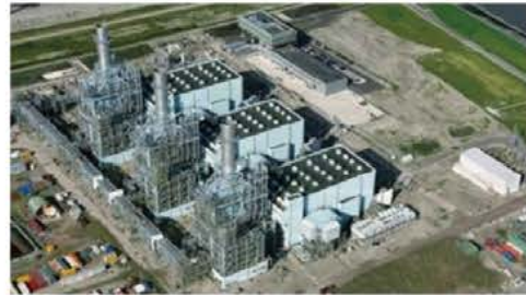
Figure 12 Vattenfall's Magnum power plant in the Netherlands
