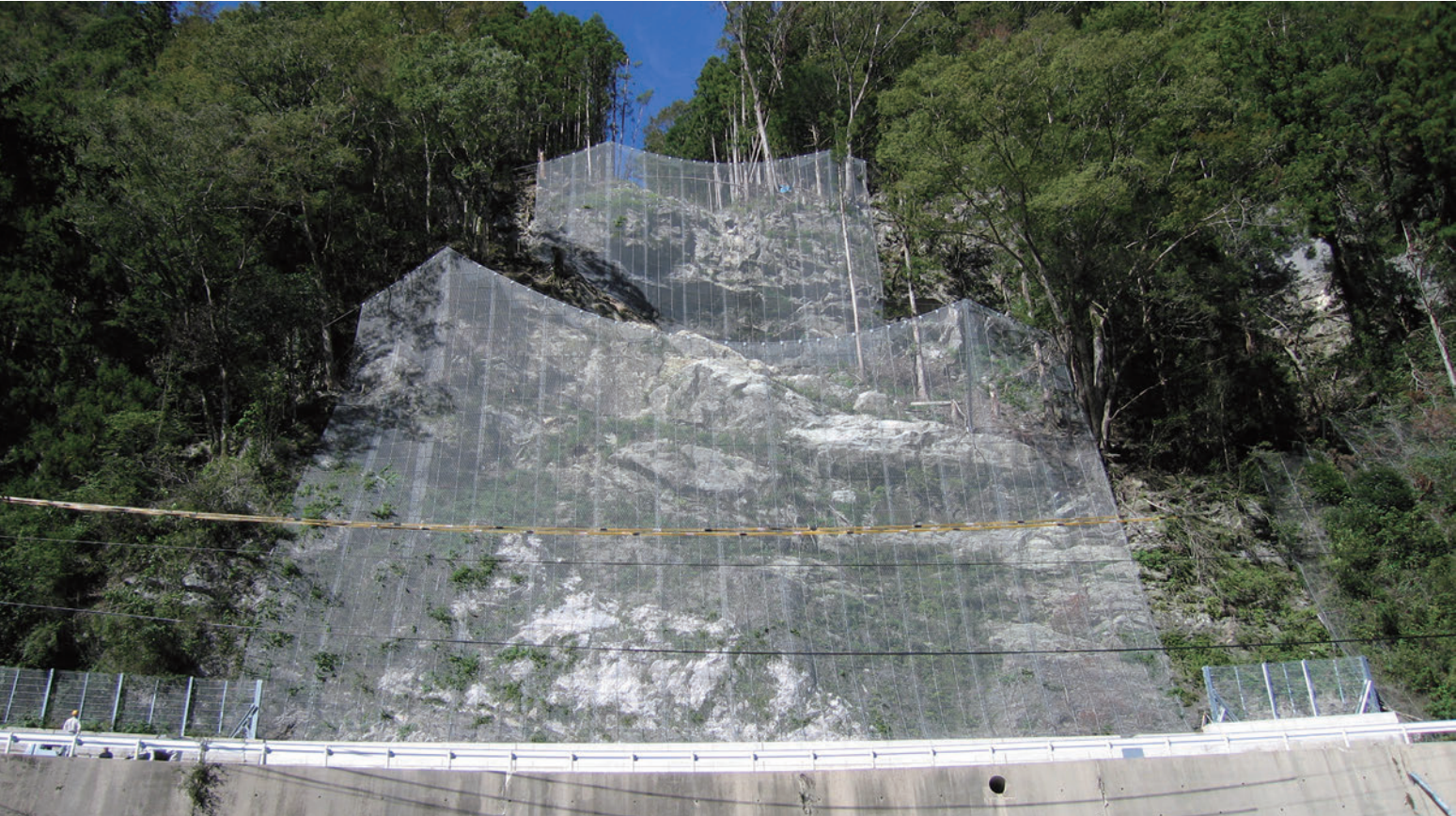
Curtain Net The construction site: Tokushima Prefecture, Japan (CN-5.0)
