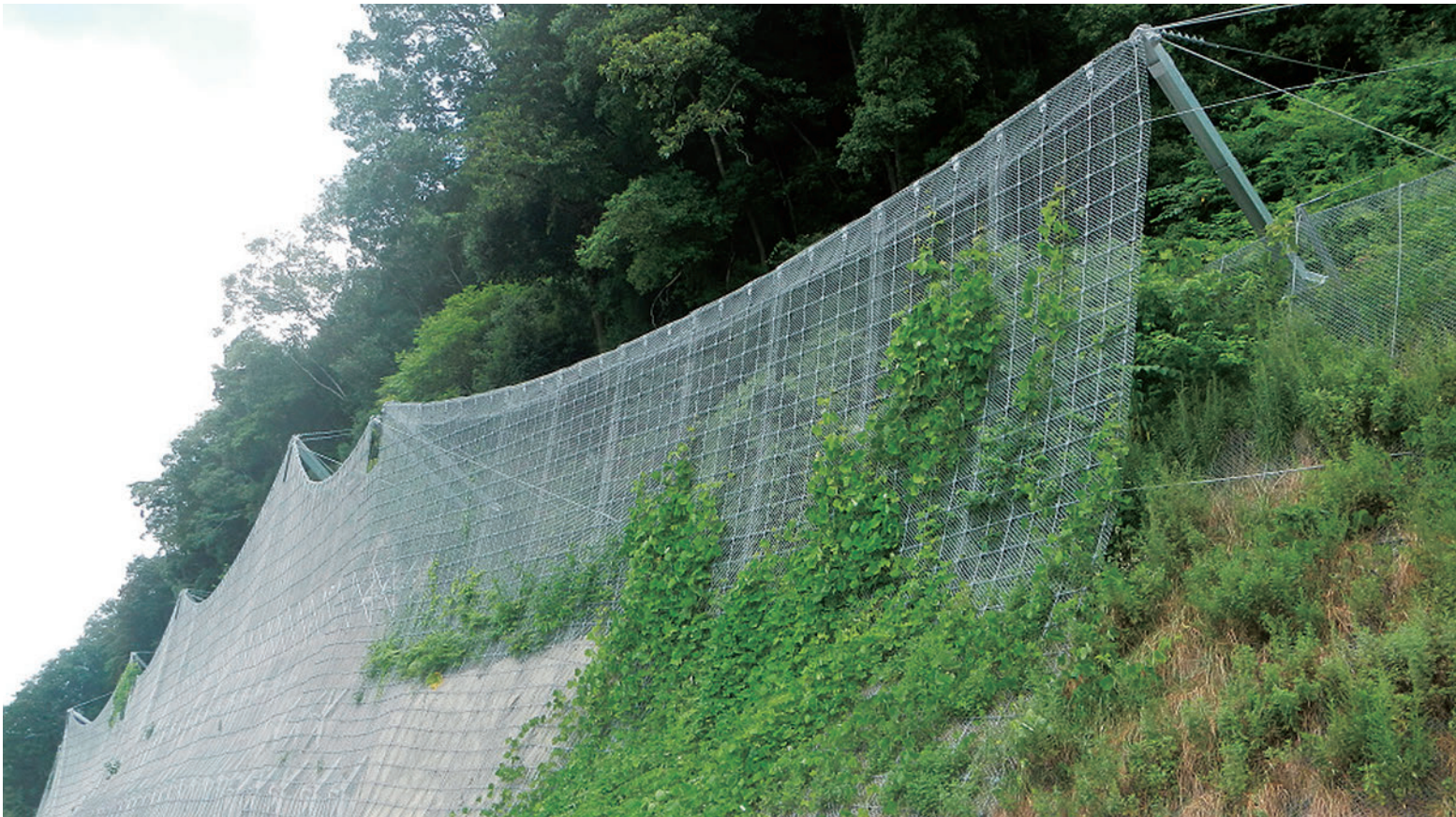
Curtain Net Super The construction site: Hiroshima Prefecture, Japan (CN-5)
