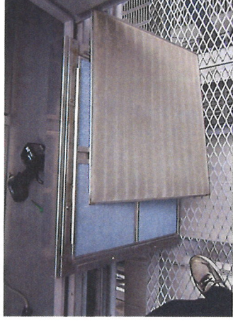
Removal of grease filter
