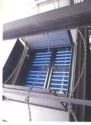
Removal of photocatalytic filter
