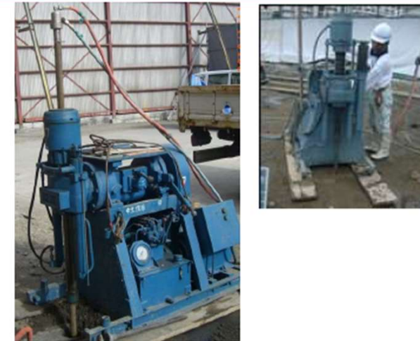
Fig. 7 Injection of RNIP into contaminated soil with chemical grouting method
