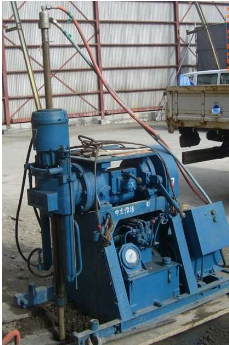
Fig. 5 Injection of RNIP® with chemical grouting
