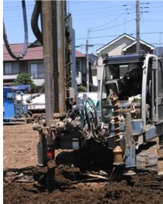
Fig. 6 Mixing of RNIP® with mechanical mixing or agitating
