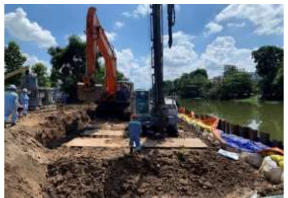
Ground improvement method is being carried out by adopting the deep mixing method.
