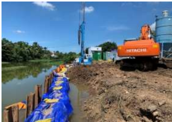
Ground improvement method is being carried out by adopting the deep mixing method.
