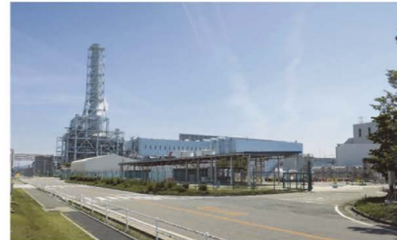
Figure 7 Construction status of Hydrogen Park Takasago (taken in May 2023)
