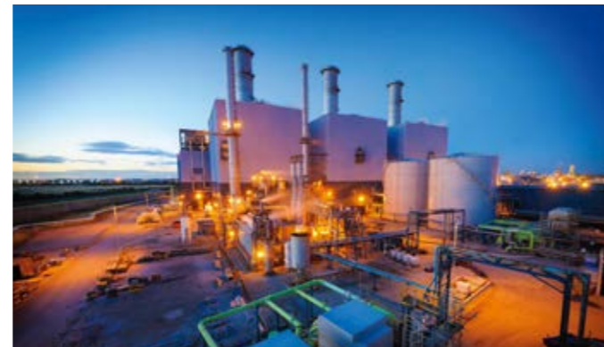
Saltend GTCC Power Plant
