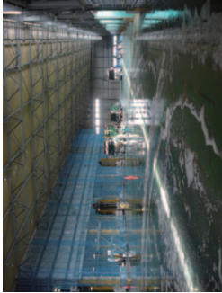
Restoration work at Kao's Sendai Logistics Center
