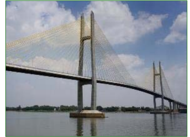
Neak Loeung Bridge, Cambodia
