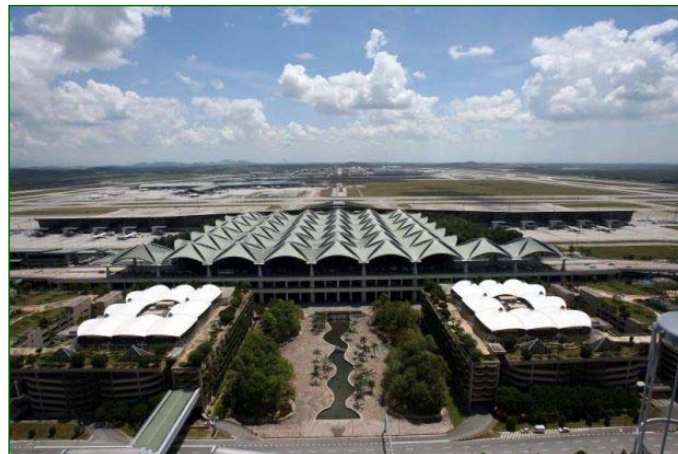
Kuala Lumpur International Airport (KLIA), Malaysia
