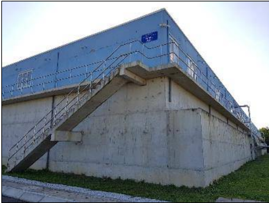
Hoa Xuan WWTP Air Blower ARS200 75KW x 6 units (2018)
