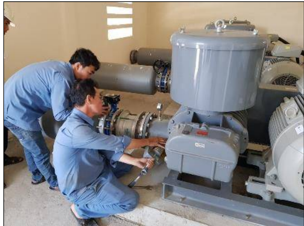
Hoa Xuan WWTP Maintenance Works
