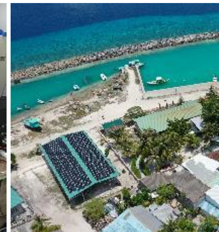
Solar PV at the project site
