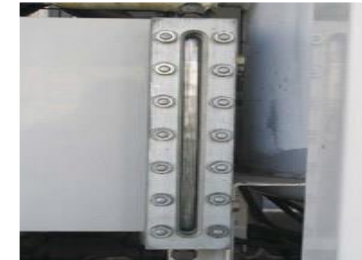
Decrease in refrigerant level
