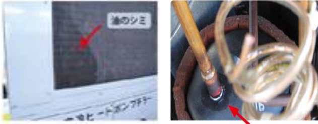
Oil leakage and stain
