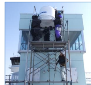
Compact size enable to install on top of existing building and to save costs and period for installation
