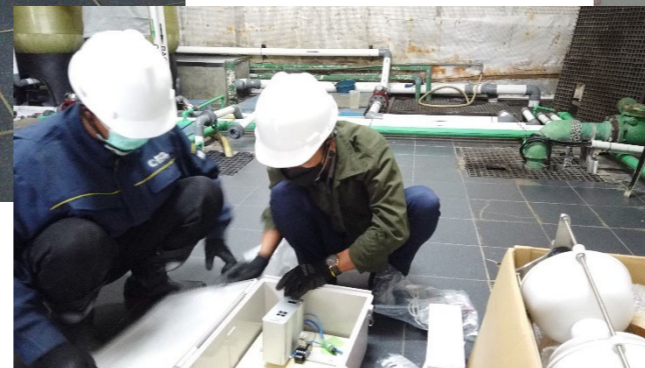
Installation of IoT monitoring system control panel
