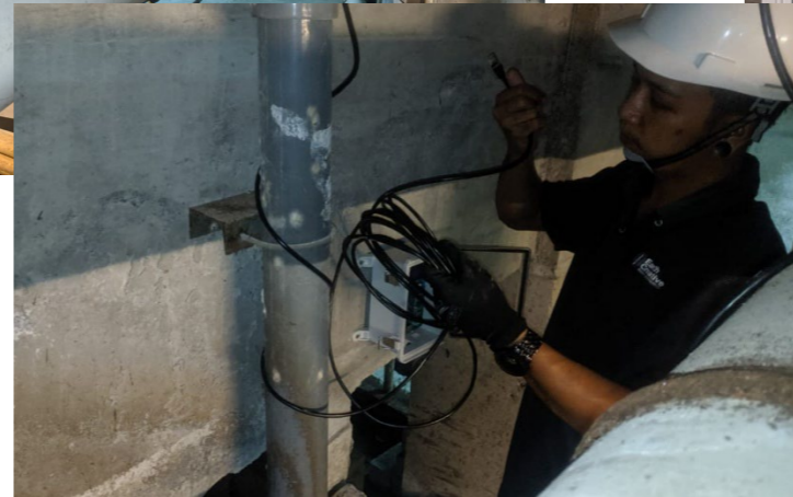
Sensor control unit and sensor connection/power supply connection
