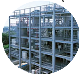
Sludge Treatment Plant
