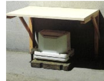
Air pump installation
