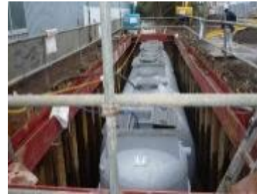
Fill a tank with water
