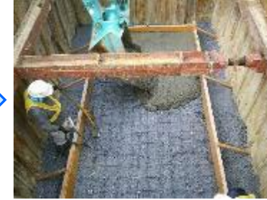
Base concrete work
