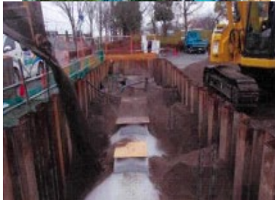
Backfilling
