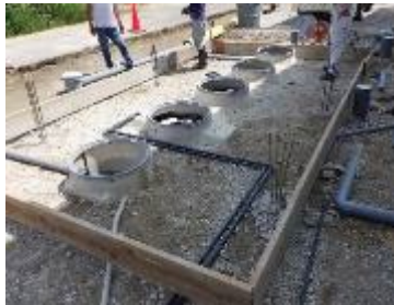
Air piping work
