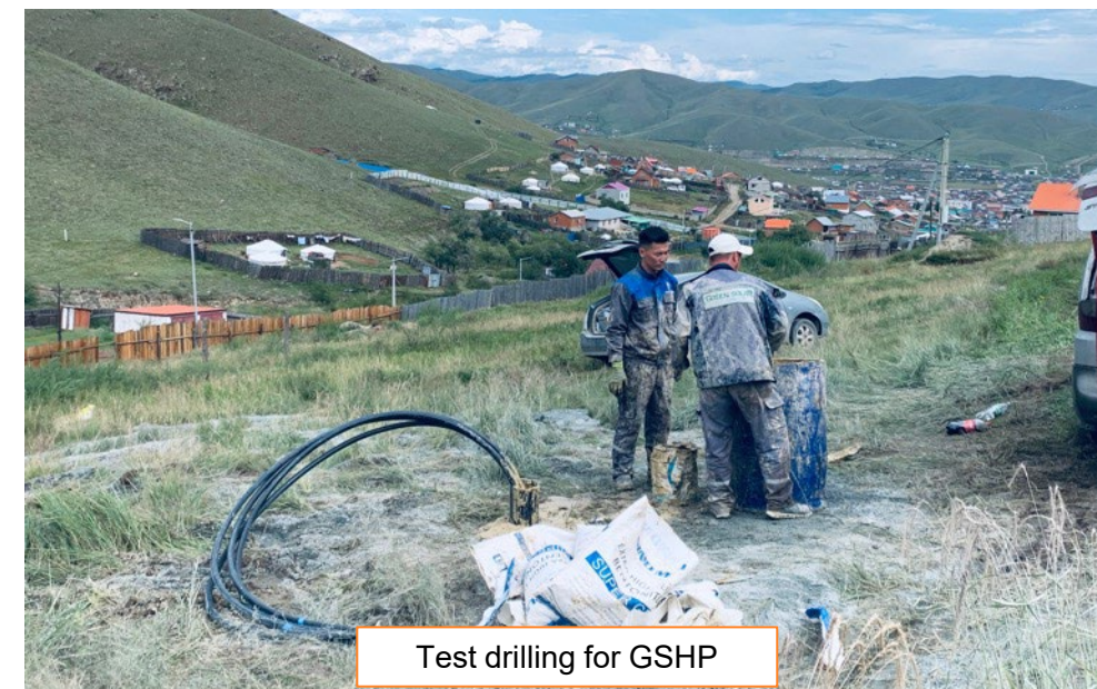
Project site for a family health center with GSHP
