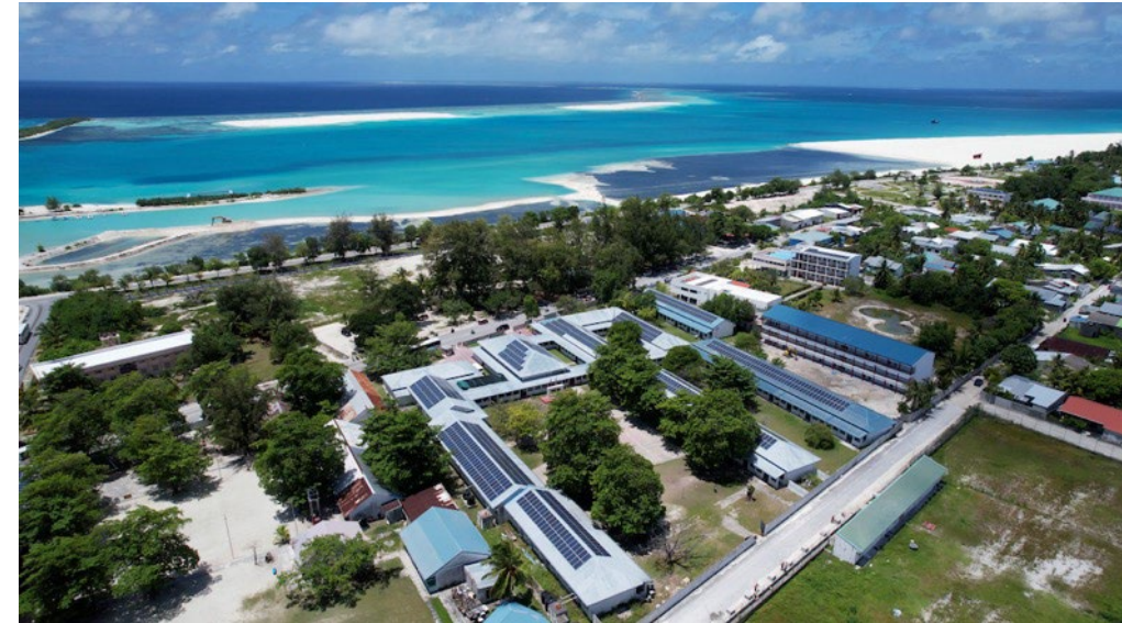
Renewable Energy Installation in Maldives
