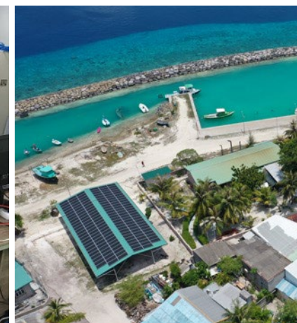
Solar PV at the project site
