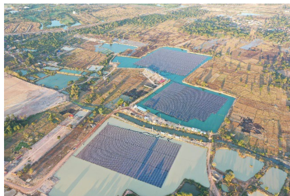
Floating Solar PV, TSB Co., Ltd., Thailand
