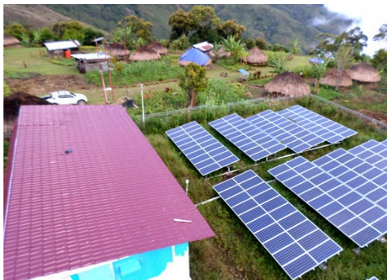
Microgrid with solar power in Indonesia
