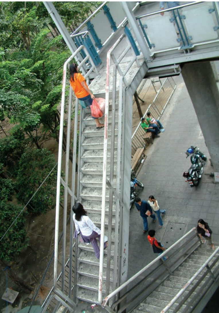
Figure 16. As shown with the steep access to this pedestrian bridge in Bangkok, infrastructure sometimes fails to account for more vulnerable users. Photo by Lloyd Wright.
