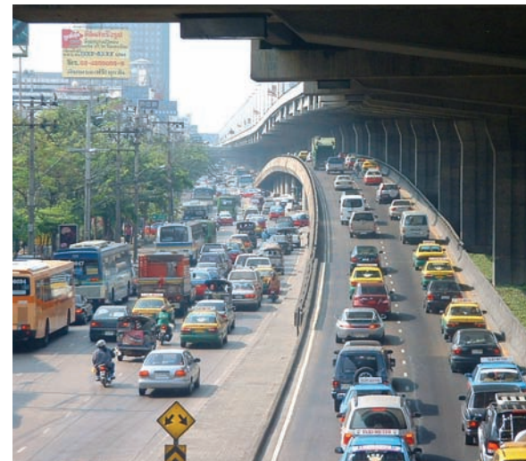
Figure 5. The myriad of flyovers and elevated roadways that dominate the landscapes of Bangkok, Delhi, Jakarta, and Shanghai has done little to relieve traffic pressures. Photo by Karl Fjellstrom.
