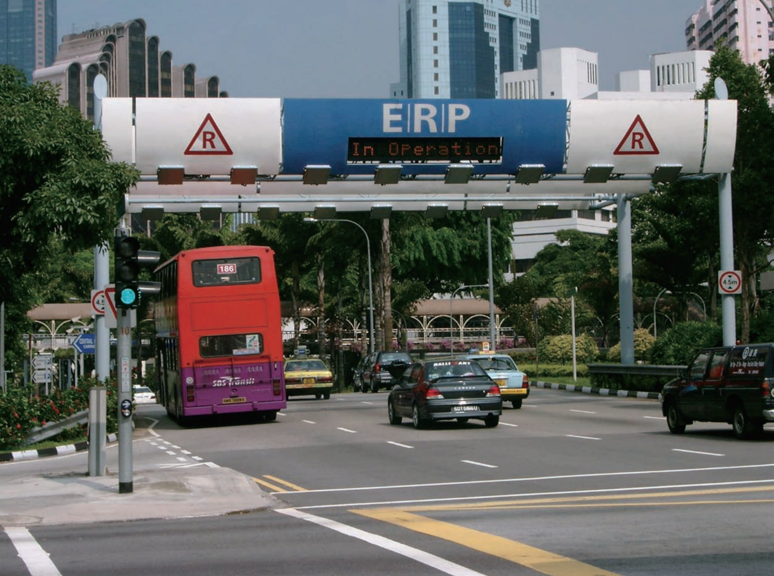
Figure 26. The Electronic Road Pricing gantry in Singapore. Photo by Manfred Breithaupt.
