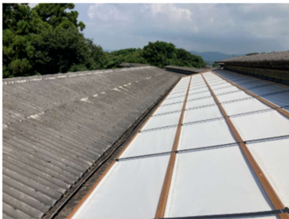
Comparison of Roof Temperatures With and Without Application of SPACECOOL
