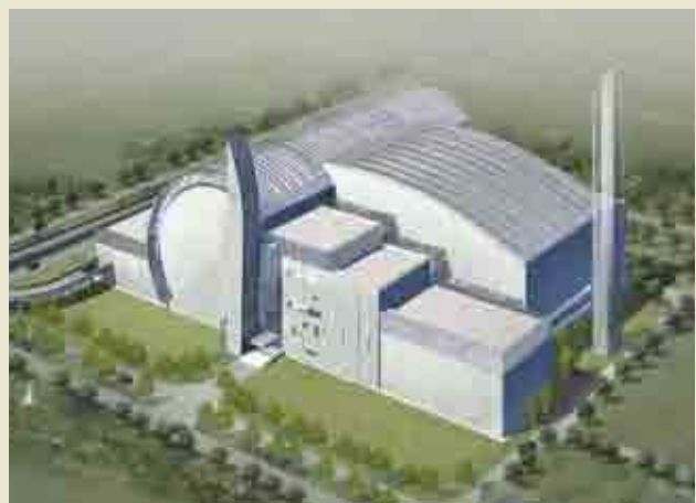
An electric generating facility with the capacity of 30,000 KW and steam condition of 4MPa and 400°C has been delivered to the incineration plant in Beijing, with capacity to handle 1,600t/day. Source: Takuma Co., Ltd.
