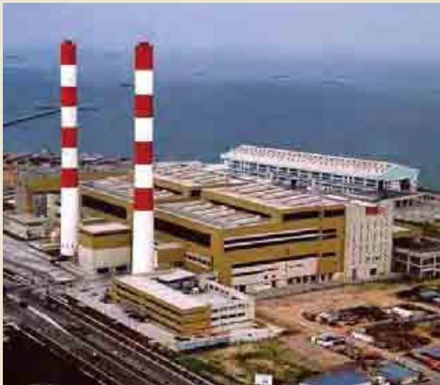
The world-largest scale plant with the capacity to handle 4,320t/day was built in Singapore in only 38 months Source: Mitsubishi Heavy Industries, Environmental & Chemical Engineering Co., Ltd.
