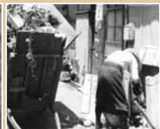
Concrete garbage box equipped in each household removed during 1960s
