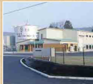
Methane fermentation and power generation facility
