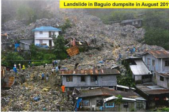
Landslide in Baguio dumpsite in August 2011.
