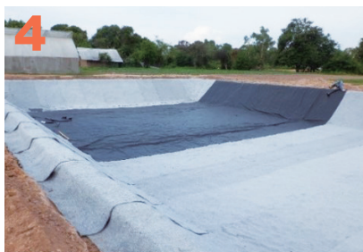
4 Lining Waterproof Sheet
