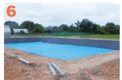
6 Floating Lid Installation
