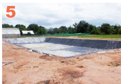
5 Waterproof Sheet Completion
