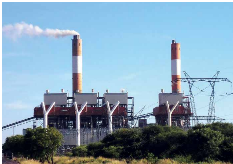
Coal thermal power plant and turbine, Botswana
