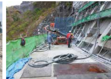
2 Anchor works for Landslides
