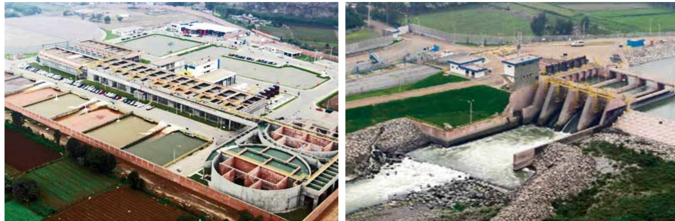
Huachipa Water Treatment Plant, Peru
