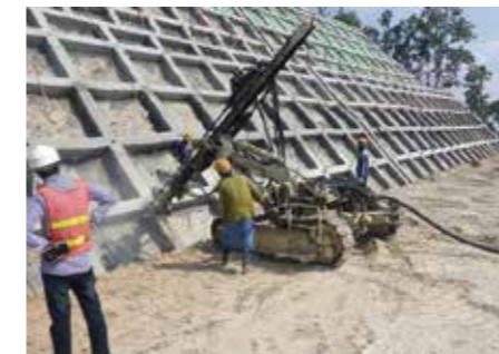
1 Crib works with rock bolt (L=3m)
