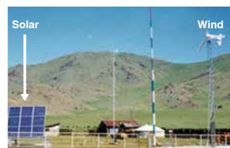
Rural Power Supply by hybrid Wind & Solar, Mongolia
