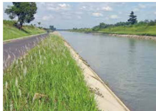
Main canal of Komenring irrigation project (59,148 ha), Indonesia
