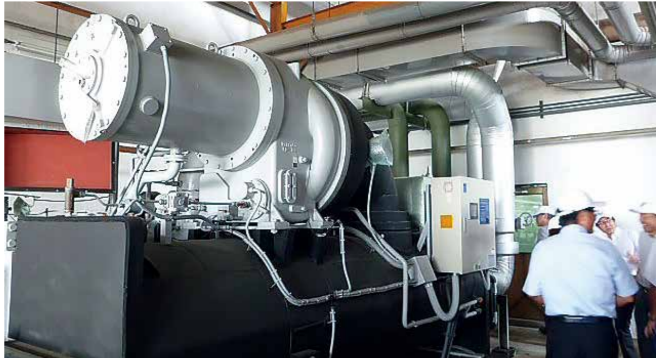
Large energy savings using high-efficiency advanced technology centrifugal chiller for factory air-conditioning, Indonesia
