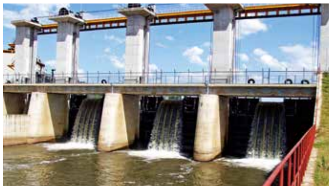
Intake weir for Sondu-Miriu Hydropower Project Kenya
