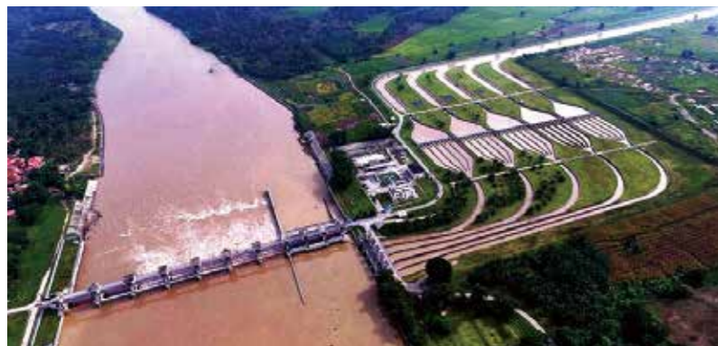
Perjaya headworks construction Stage I, Indonesia
