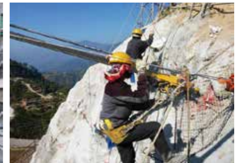
3 High intensity Net with rock bolt for erosion control
