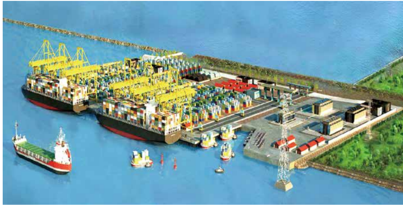
Lach Huyen Port Construction Project, Vietnam (on-going) (source: JICA study report)
