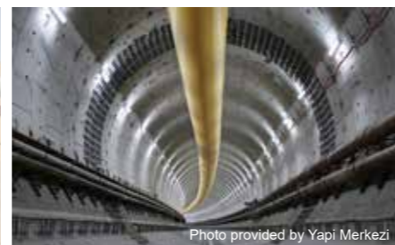
Bosphorus Straits (Marmaray) Shield Tunnel, Turkey
