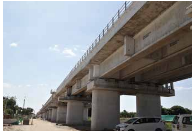
Western Dedicated Freight Corridor Project, Delhi-Mumbai, India Viaduct with PSC girders span of 56 x 19.8m for WDFC
