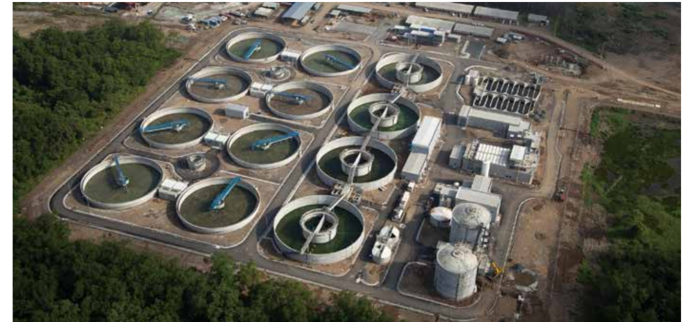
Juan Diaz Wastewater Treatment Plant, Panama City and Bay Sanitation Project, Panama
