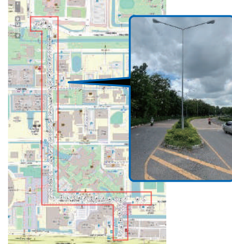
Our smart LED streetlights were installed on the campus
