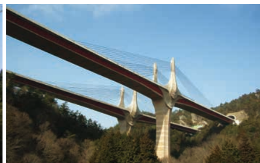
Left: Basic and Detailed Design of Yatogawa Bridge, PC5 span continuous corrugated steel web box girder bridge (Japan)
