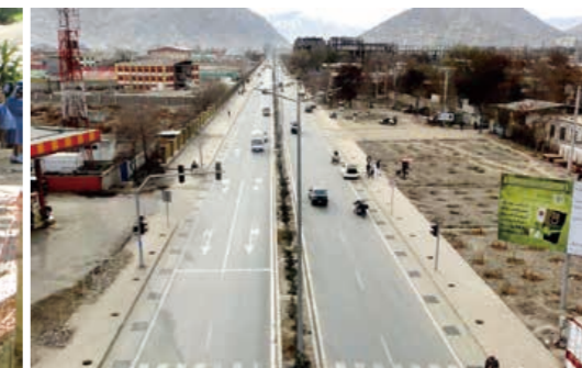
Left: Project for Improvement of Urban Roads and Drainage for Reconstruction of Leogane (Haiti)
