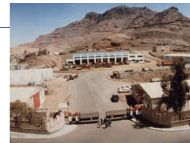
1993 Construction Machinery Training and Maintenance Center (Yemen)
