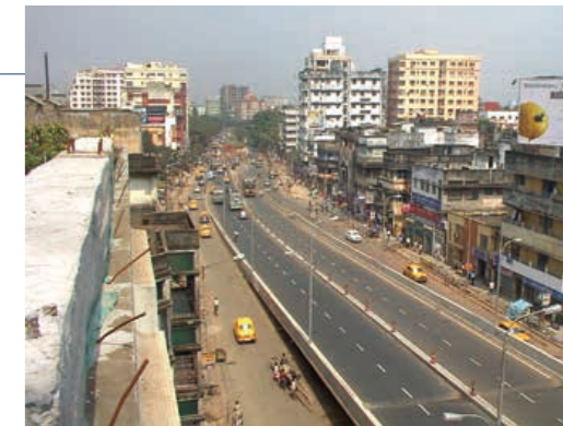
1997 Kolkata Transport Infrastructure Development Project (India)
