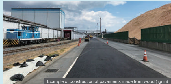
Example of construction of pavements made from wood (lignin)
