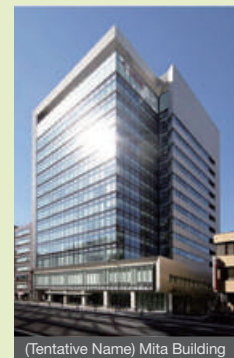
(Tentative Name) Mita Building
