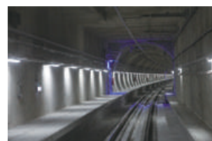
Bosphorus Tube Crossing Railway Tunnels and Station, Istanbul
