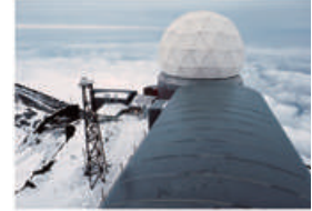
Mt. Fuji Summit Radar Site
