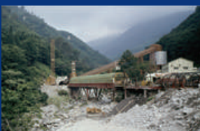
Joetsu Sinkansen Line Daishimizu Tunnel
