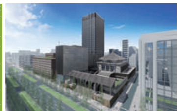
(Tentative name) Honmachi 4-Chome Project (Osaka-shi, Osaka) Owner: Taisei Corporation and Soai Gakuen * Joint development project
