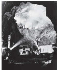
Kansai Electric Power Co., Inc., Kurobegawa No.4 Hydropower Plant [5th segment]
