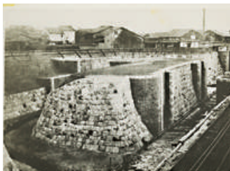
Lake Biwa Canal Sluice Gate
