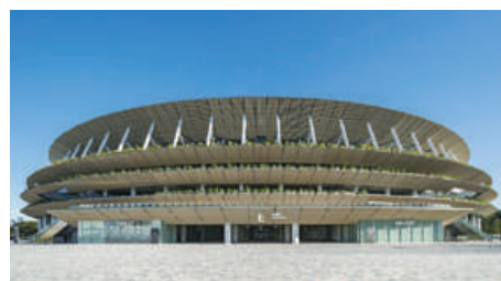
Japan National Stadium
