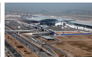
Noi Bai International Airport 2nd Passenger Terminal, Hanoi, S.R. Vietnam
