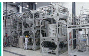
Construction of Takasago Chemical iFactory (Kakegawa-shi, Shizuoka) Owner: Takasago Chemical Corporation
