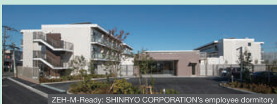
ZEH-M-Ready: SHINRYO CORPORATION's employee dormitory
