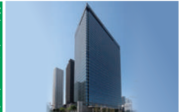
New Building Construction Work for Nishi-Shinjuku 5-chome Kita Project (Shinjuku-ku, Tokyo) Owner: Business Association of Nishi-Shinjuku 5-chome North Block Disaster Prevention Improvement Project
