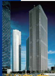
Shinjuku Center Building
