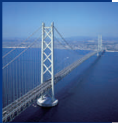
Kobe Awaji Naruto Expressway Akashi Kaikyo Bridge 3P [substructure part 2]
