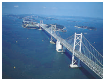
Minami & Kita Bisan-Seto Bridges [substructure, North segment]
