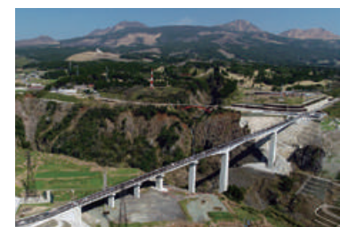
National Highway 325, Shin-Aso Ohashi Bridge
