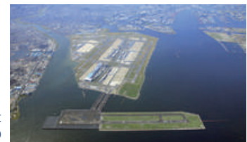
Tokyo International Airport Runway D
