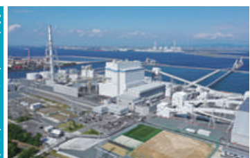
Taketoyo Thermal Power Station Unit 5, Civil Engineering & Building Construction Work (Chita-gun, Aichi) Owner: JERA Power TAKETOYO LLC.
