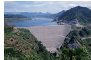
Cirata Hydroelectric Power Plant, Indonesia
