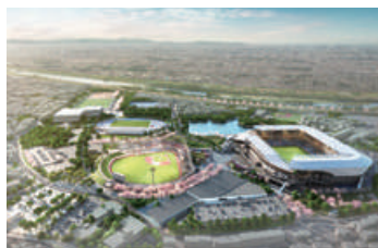
Construction for Todoroki Green Space Redevelopment, Operation, Etc. Project (Kawasaki-shi, Kanagawa) Owner: Kawasaki Todoroki Park Co., Ltd.
