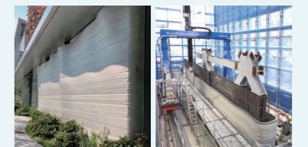
View of the whole wall 3D printing construction
