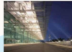
2007 Changi Airport Terminal 3 (Singapore) The method of lifting up steel frame trusses measuring 300 meters wide and 215 m deep, was a first in the world
