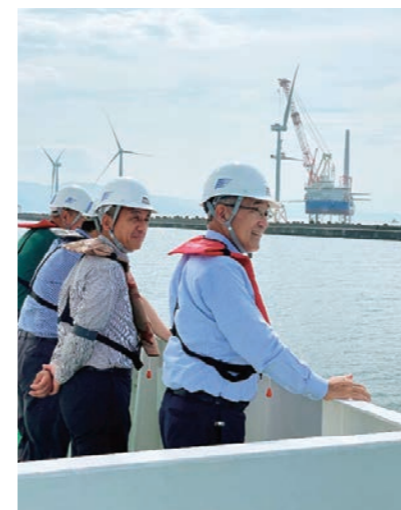
Touring offshore wind farm generation facility construction site
