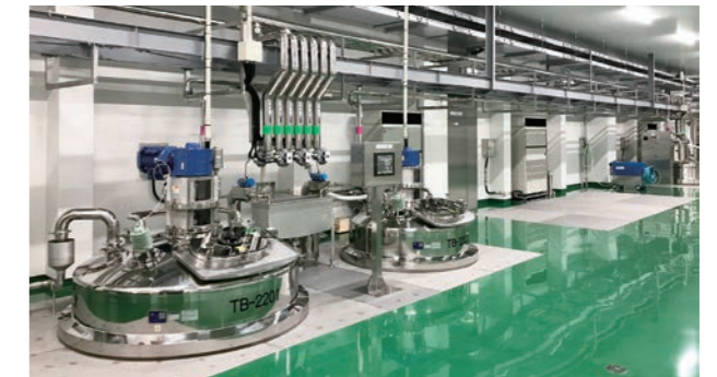
Yamasa Corporation Shiga Ryuo Plant Manufacturing tanks and automatic raw material supply equipment (Gamo County, Shiga)
