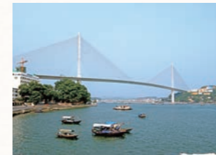
2006 Bai Chay Bridge (Vietnam) A giant 903-meter cable-stayed bridge over a World Heritage Site
