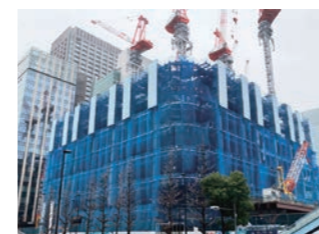
Nihonbashi 1-chome Naka-area, pillar-front curing (Chuo Ward, Tokyo)
