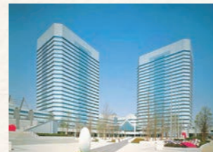
1990 Makuhari Techno Garden Large-scale intelligent building complex with an advanced building management system and R&D functions forming the core of the Makuhari New City Center Project
