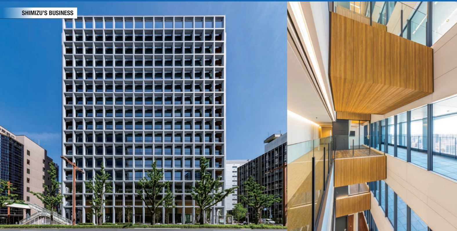
Nagoya Shimizu Fukoku Seimei Building (Nagoya, Aichi) Front of the building
