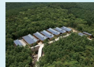
2013 SEICHO-NO-IE "Office in the Forest" Japan's first ZEB realized through energy conservation and energy creation
