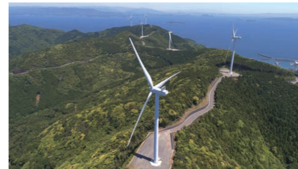
Hirado-Minami Wind Power Plant South Site (Hirado City, Nagasaki)
