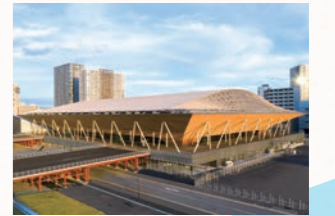
2019 Ariake Gymnastics Centre One of the world's largest timber-framed roofs. Designed to communicate the Japanese culture of using wood and sustainability.
