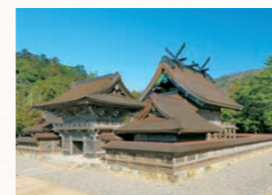
2013 Izumo Taisha Shimizu was in charge of preservation and repair work on 14 buildings during the renewal of the Izumo Grand Shrine for the first time in 60 years.
