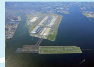
2010 Tokyo International Airport D-runway Large-scale offshore runway featuring hybrid structure of reclaimed land and pier, uncommon around the world (photo courtesy of Haneda reexpansion D runway JV)
