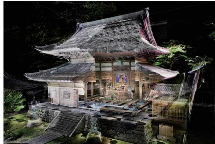
Point cloud data of main hall (both exterior and interior displayed simultaneously)
