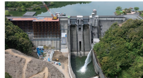
Nomura Dam construction (Seiyo City, Ehime)
