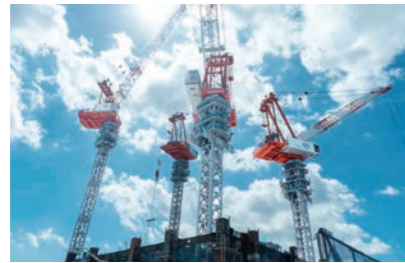
Rental Large Tower Crane
