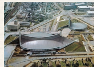
1964 Main Gymnasium of the National Indoor General Stadium Unprecedented wire-suspended roof structure
