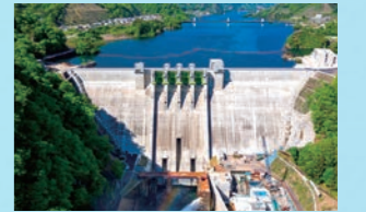
2020 Yamba Dam The Company's first dam exceeding 100 meters in height. The active use of pre-cast and ICT substantially shortened the construction period.
