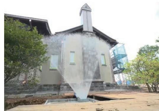
Jiu system spraying water onto a building
