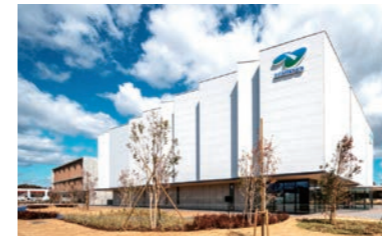
Tsuchiura Techno BASE (Tsuchiura City, Ibaraki)
