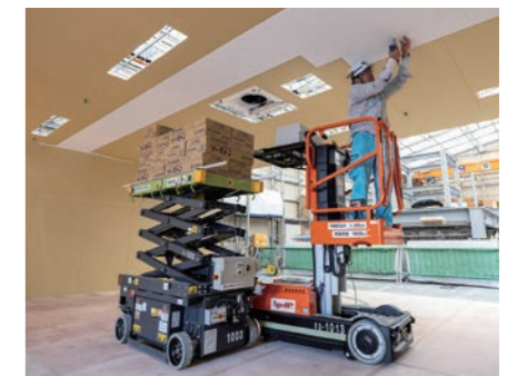
Ceiling finishing work using Sky Runner (right) and Sky Table (left)
