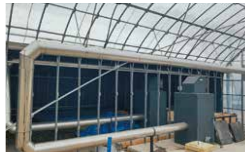
Chimney installation (maximum 20m) By pulling the chimney horizontally, the inside of the house can be heated efficiently.
