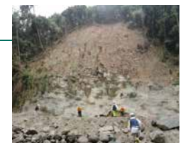
▲ An on-site field survey of collapsed land
