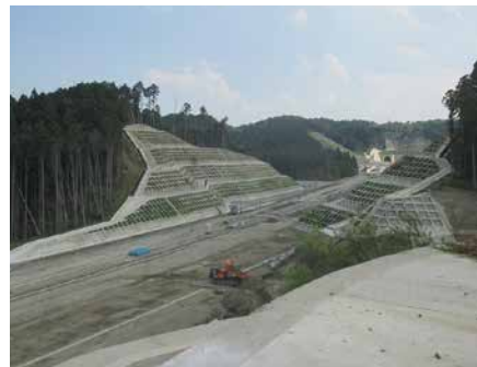
▲Shin-Meishin Expressway while under construction (Shin-Yokkaichi Junction to Komono) Opened in March of 2019
