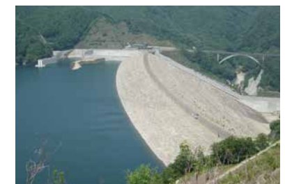
▲ A dam project utilizing CM
