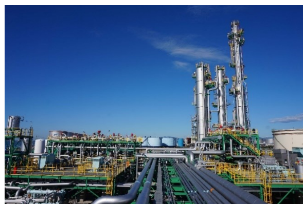
Tomakomai CCS Demonstration Project Center
