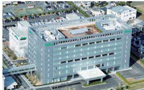
Nidec Shiga Corporation Technical Center
