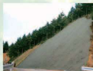
③ Just after installation of SP-45
