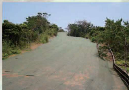
② Just after construction
