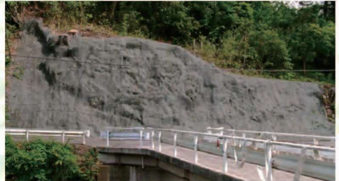
② Just after construction
