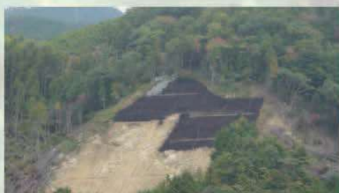
① Under construction of SP-45 after seed and soil spraying
