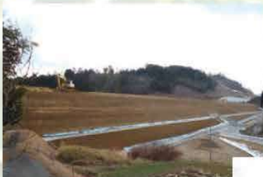
① Before construction
