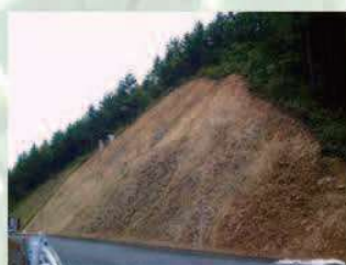
① Before construction
