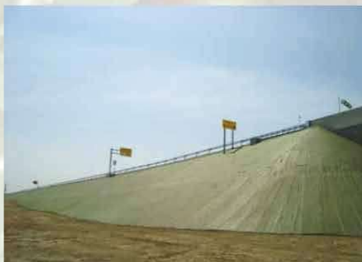
Just after construction
