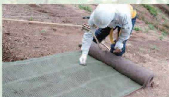
③ Fixed on the slope surface
