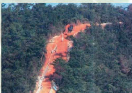
① Before construction
