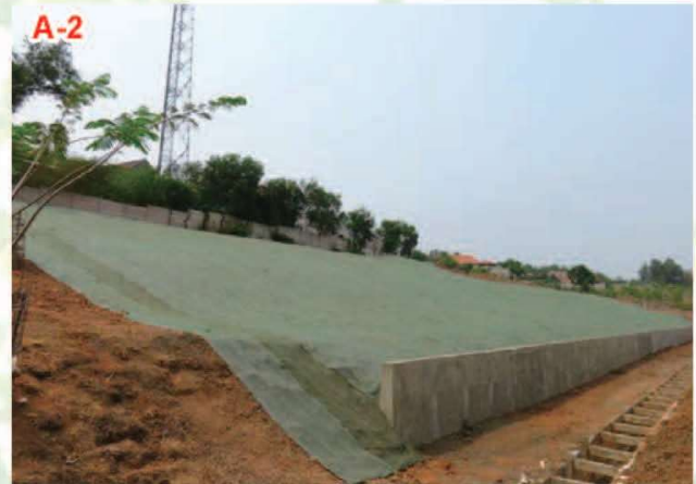
① Just after construction
