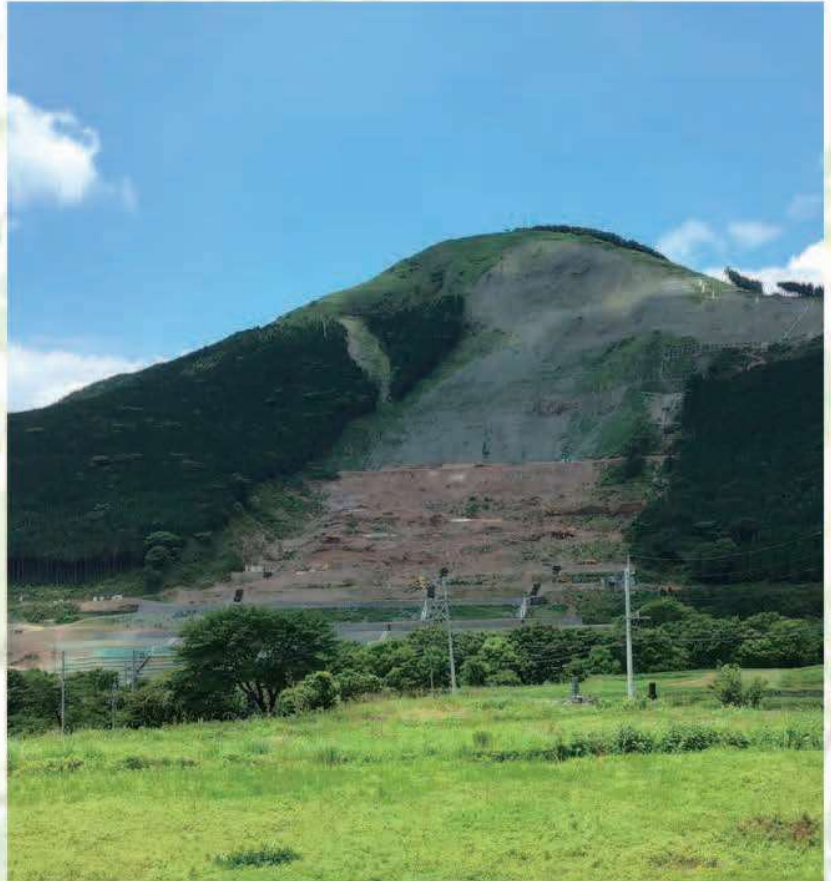
③ 1 year and 8 month after construction start
