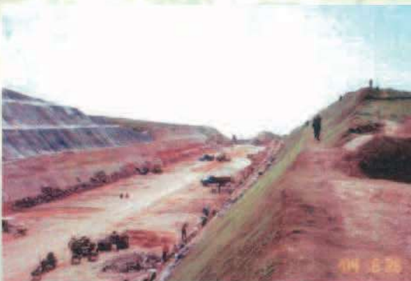
① Under construction
