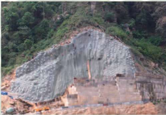
② Under construction
