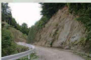
① Before construction
