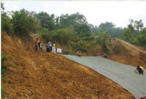
② Just after construction
