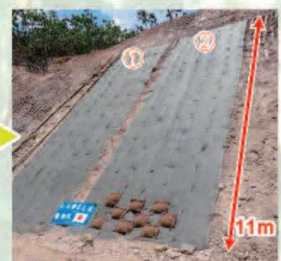
③ Just after construction
