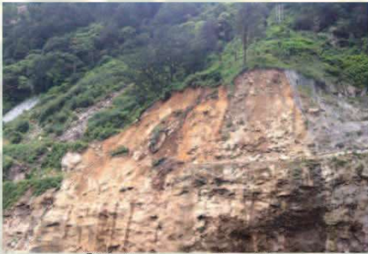
① Before construction
