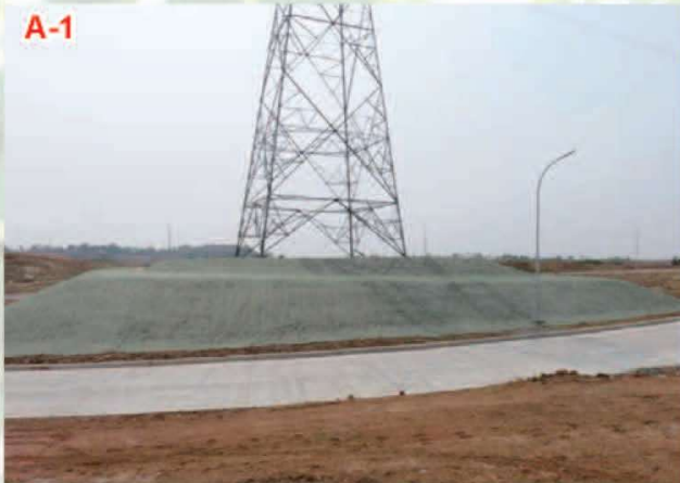
① Just after construction
