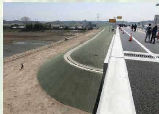
Just after construction
