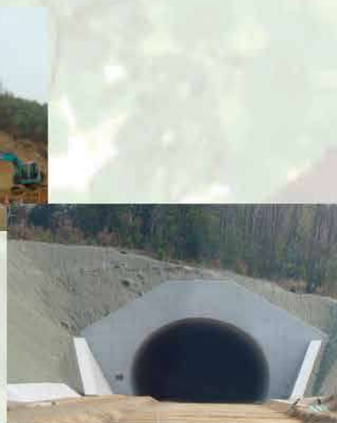
② Just after construction
