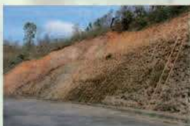
① Before construction
