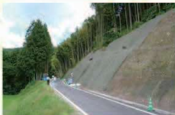
① Under construction
