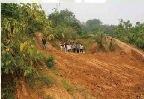
① Before construction
