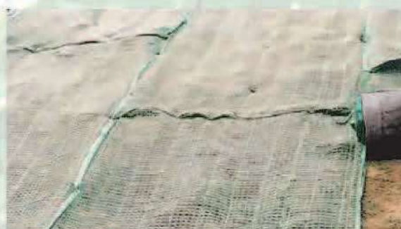
④ Several sheets laid and fixed at the overlaps
