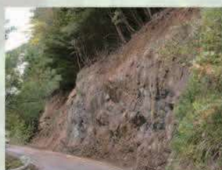
① Before construction
