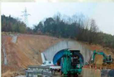
① Before construction
