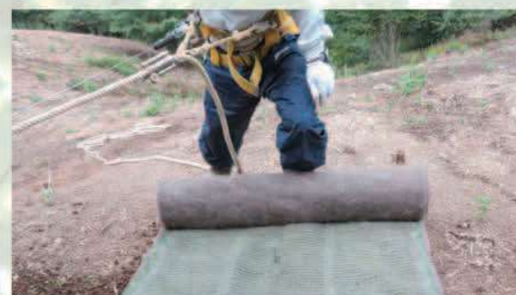
② Covered on the slope surface
