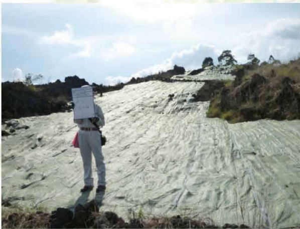
① Just after construction
