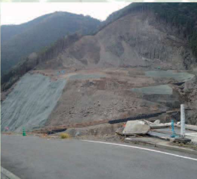
① 4 months after construction start
