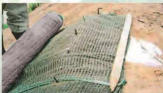
① Fixed on the top of slope shoulder
