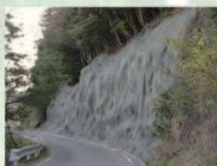
② Just after construction
