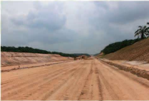
① Before construction
