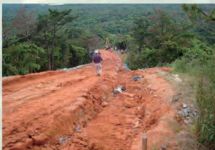
① Before construction
