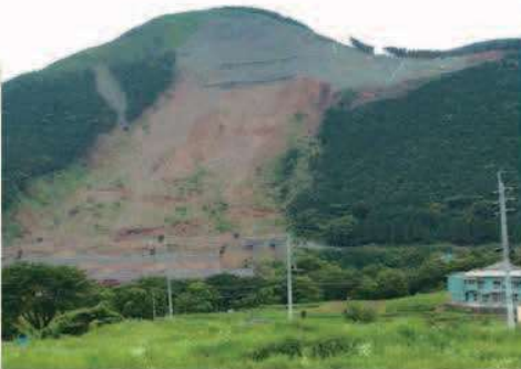
② 8 months after construction start
