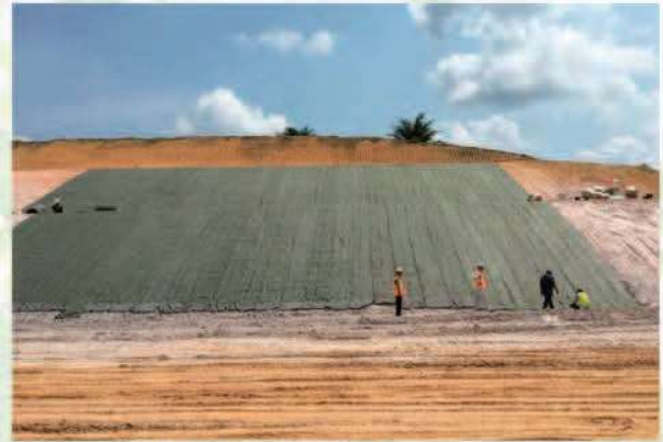
② Just after construction
