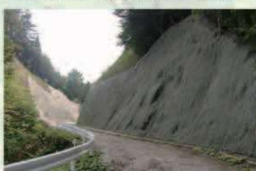
② Just after construction
