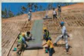
② Under construction
