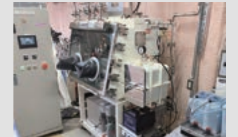
Formic acid production facilities
